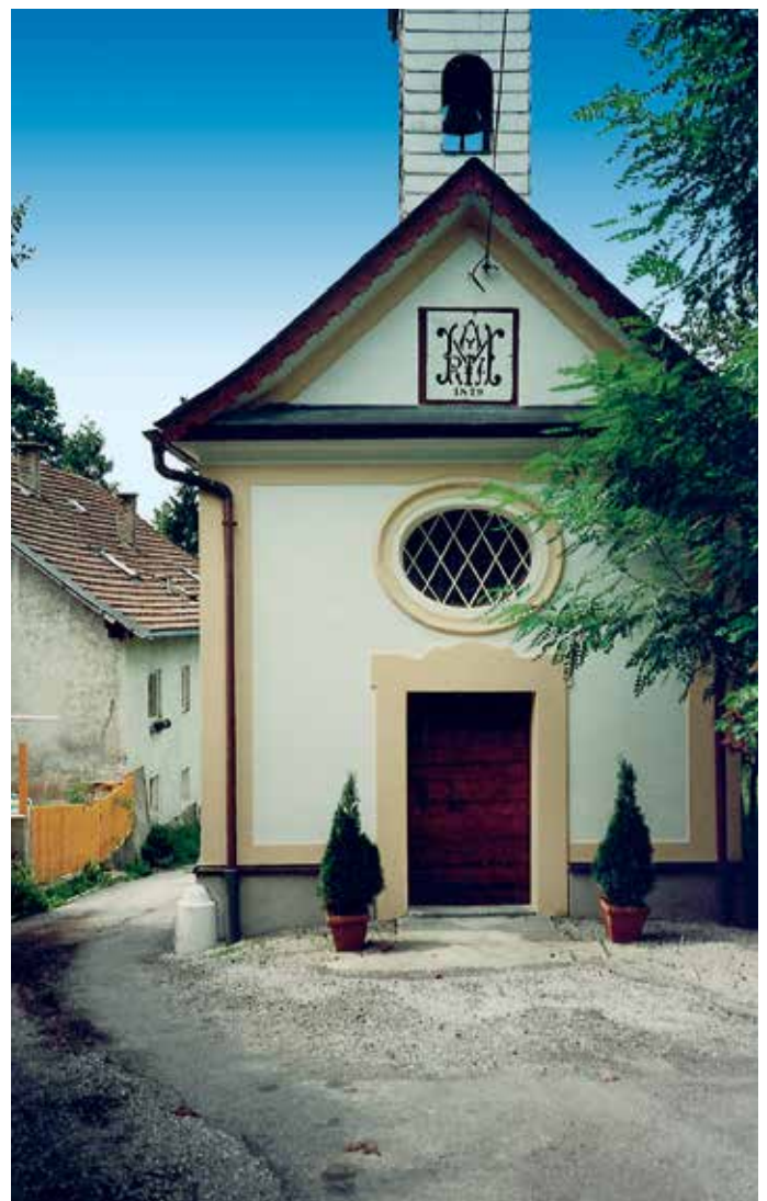
Figure 1: Successful reconstruction of a chapel in Gnigl (municipal district of Salzburg, AT). With special plaster systems even damp brick-work can be reconstructed in a way which makes it protected durably against further negative influences of humidity. © maxit
