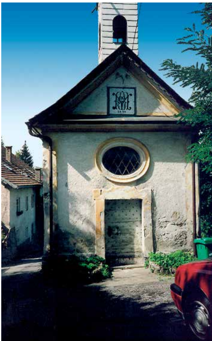
Figure 1: Successful reconstruction of a chapel in Gnigl (municipal district of Salzburg, AT). With special plaster systems even damp brick-work can be reconstructed in a way which makes it protected durably against further negative influences of humidity. © maxit
