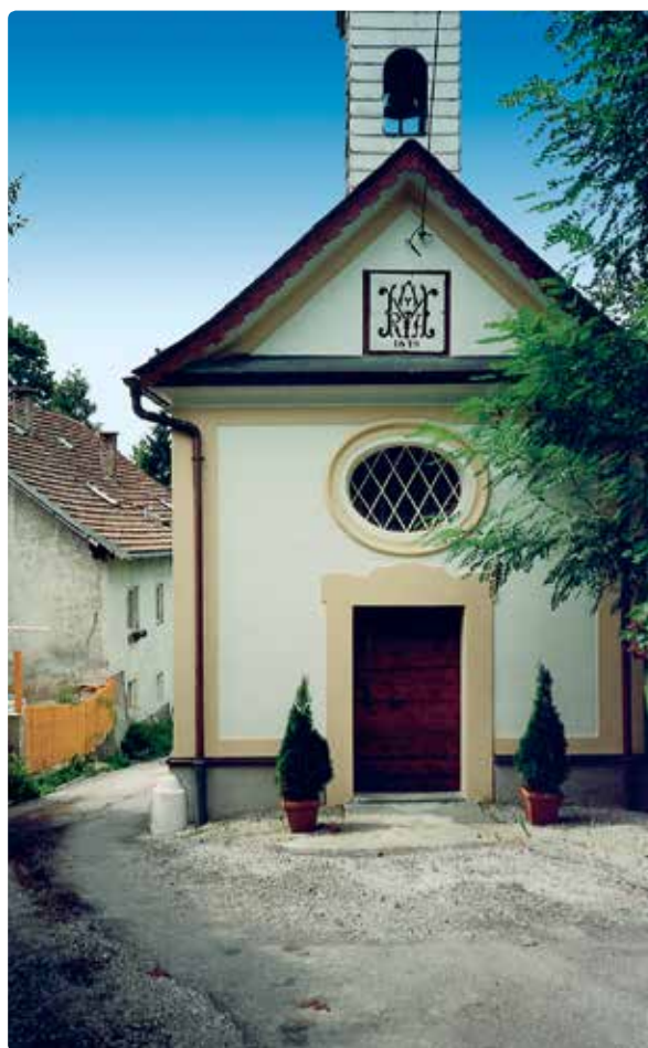
Fig. 1: Successful reconstruction of a chapel in Gnigl (municipal district of Salzburg, AT). With special plaster systems even damp masonry can be reconstructed in a way which ensures a durable protection against further negative influences of moisture.
