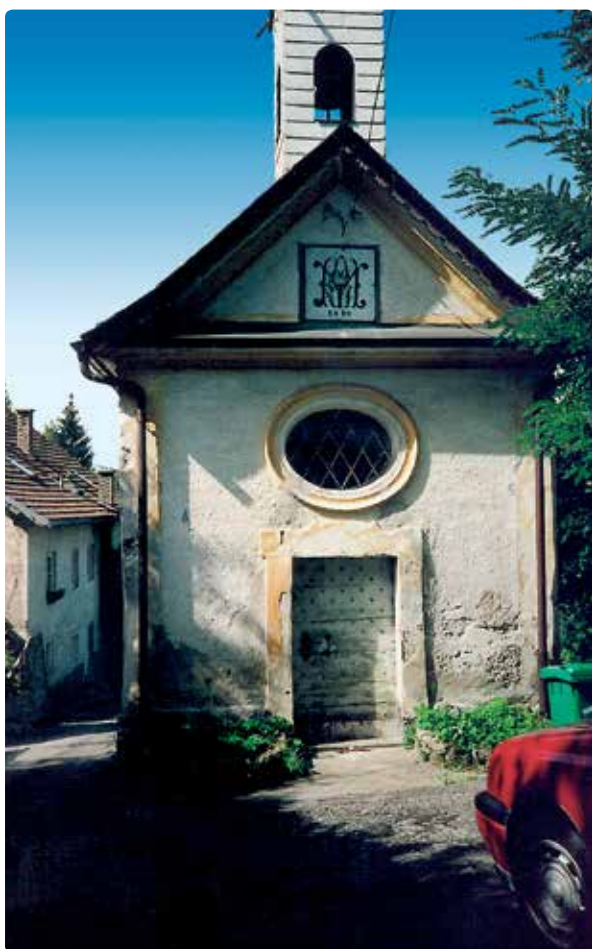
Fig. 1: Successful reconstruction of a chapel in Gnigl (municipal district of Salzburg, AT). With special plaster systems even damp masonry can be reconstructed in a way which ensures a durable protection against further negative influences of moisture.
